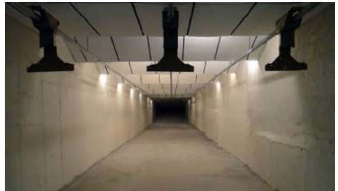
Underground Firing Range
